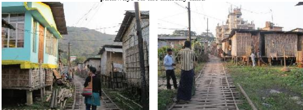
Image 1 (left). Bhootnath Milanpath Dolki: Houses on stilts Image 2 (right). Bhootnath Milanpath Dolki: Bamboo weaves used to make pathways on the marshy land
