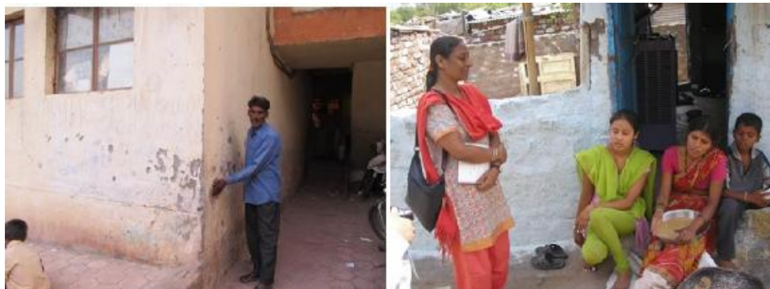
Figure 13: A resident showing the bad quality of plaster (left) and transit housing residents raising their concerns (right)
