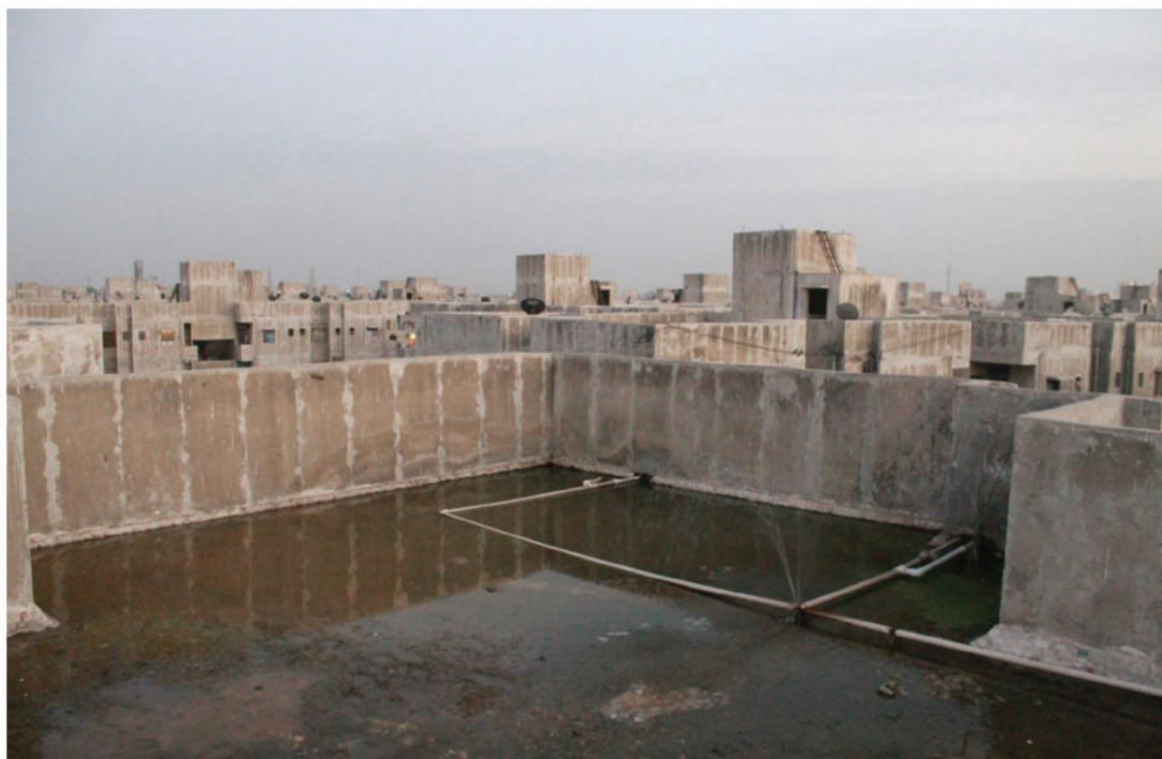
Leakages and a pipe burst on the terrace of one of the buildings in Sadbhavna Nagar – this drains out the water from the overhead water tank due to which the building's residents cannot get 24-hour running water supply (this condition of water pipes is commonly seen on the terraces of many of the buildings)
