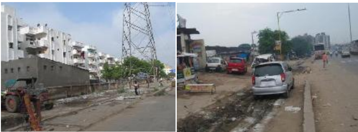
Figure 12 (Left) An electricity transmission pylon obstructing the NMT lane (Right) The sorry state of NMT lane
