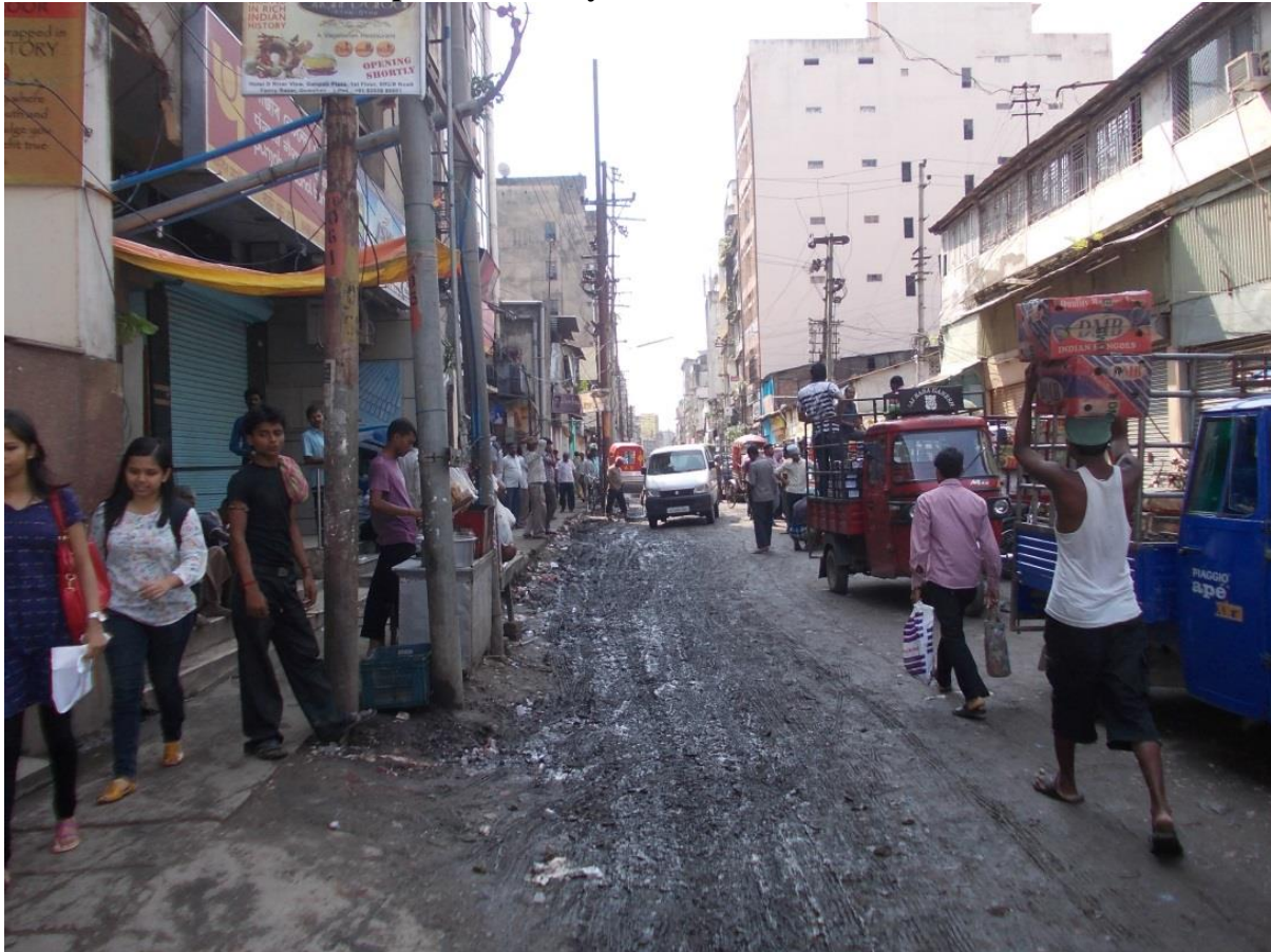
Picture 3: Encroached footpaths in Fancy Bazar area
