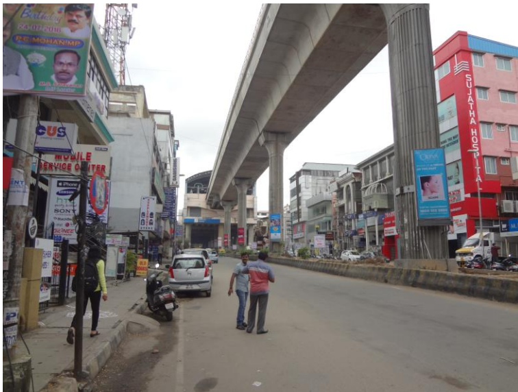
Figure 19: MG road metro station, Bengaluru
