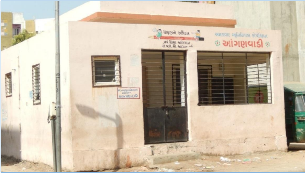
Figure 9: Functioning anganwadi at the Balol Nagar site
