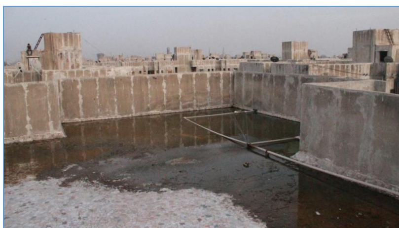
Figure 16: Water pipes leaking on a building's terrace, Sadbhavna Nagar
