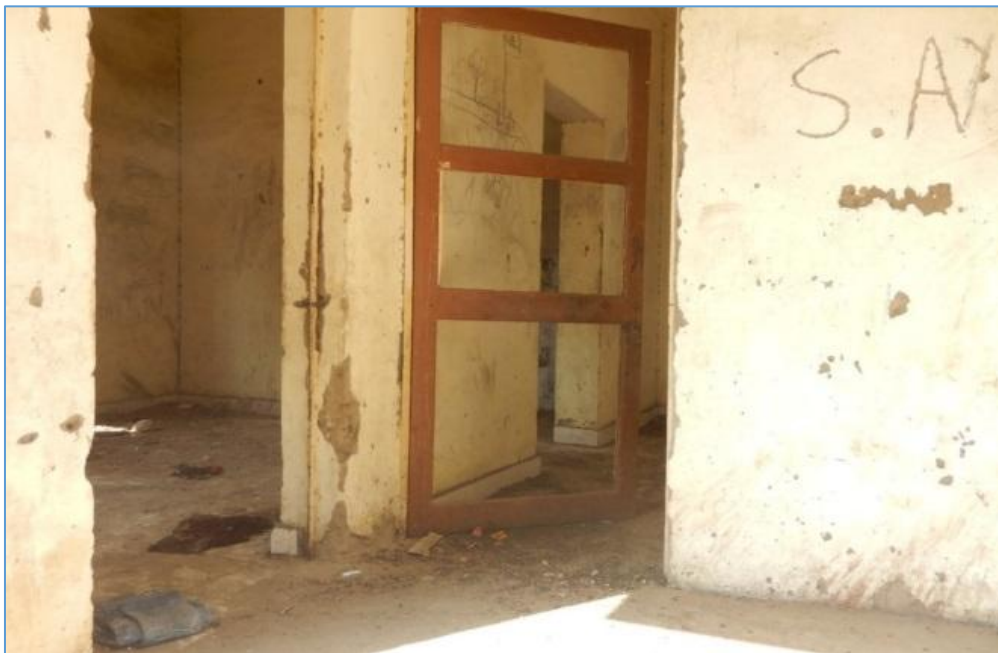
Figure 13: Vacant health sub-centre at Makrand Desai Nagar
