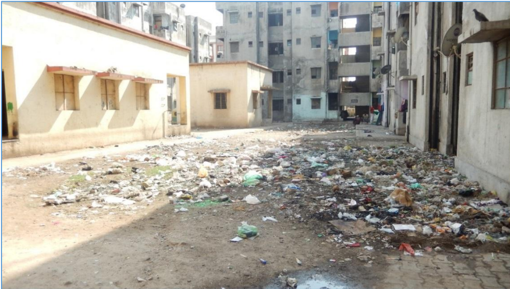
Figure 18: Indiscriminate dumping of waste by residents in common areas of the site at Sadbhavna Nagar
