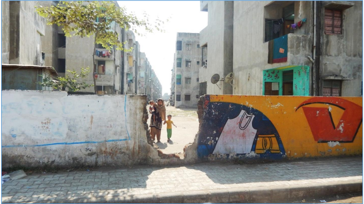
Figure 7: Sadbhavna Nagar, BSUP site at Vatwa
