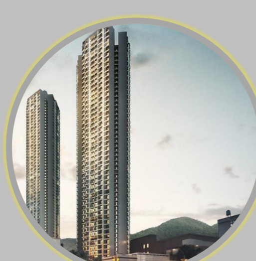
Residential Project, Maharashtra
