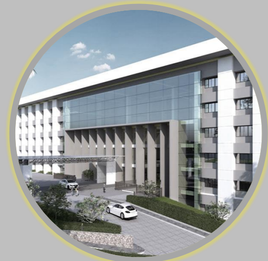
Hospital Project, Kerala
